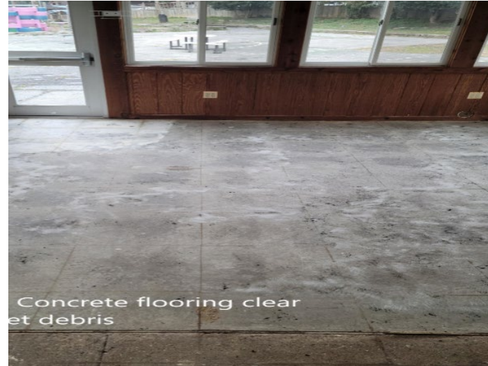
Removal of Carpet in Future Kitchen/Cafeteria
