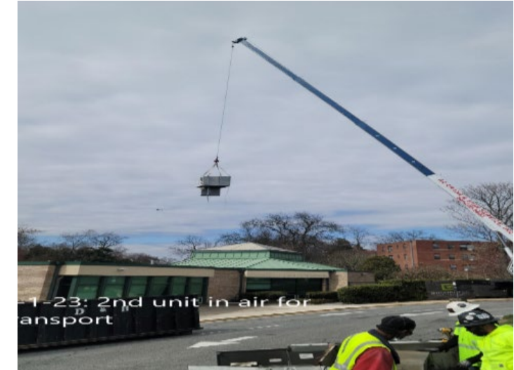
Removal of RTUs for Kitchen/Cafeteria HVAC
