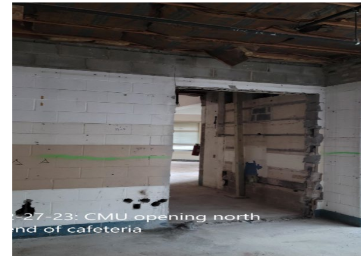
CMU Demolition Progress
