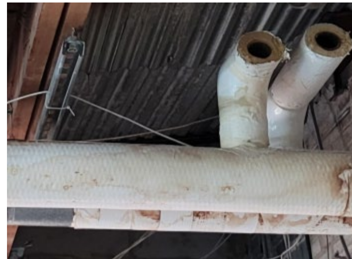
HVAC Demolition Progress
