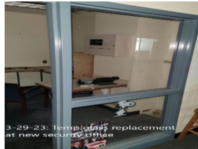
Damaged glass replacement
