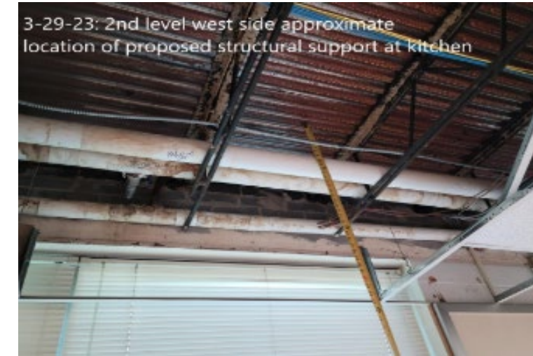
Assessment of proposed structural support took place
