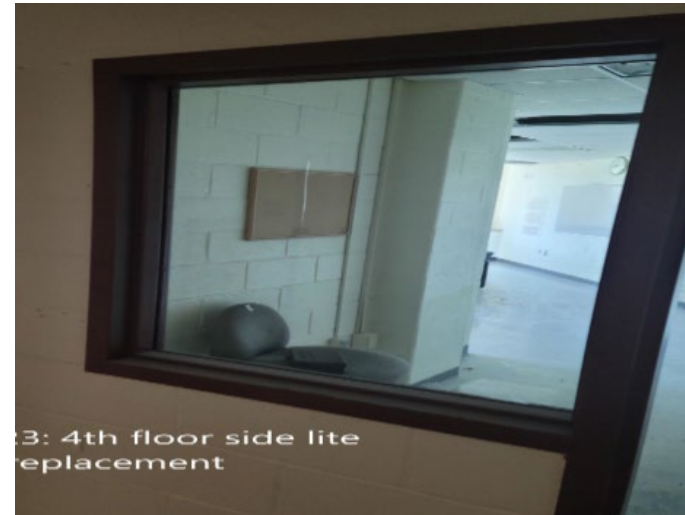
Damaged Glass replacement began in building
