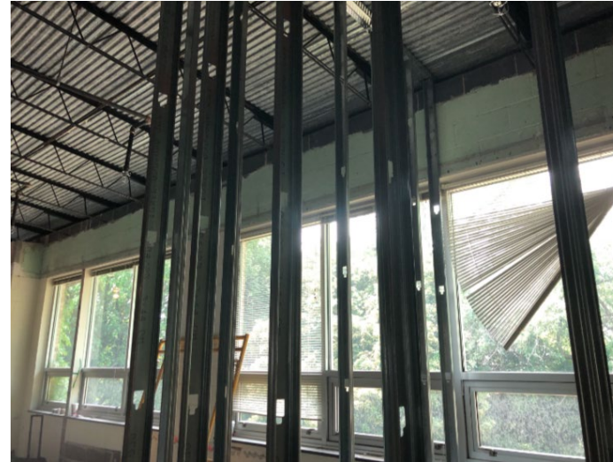
Wall framing in kitchen
