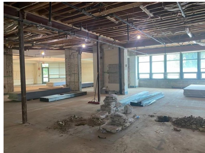
Flooring work to accommodate rough-ins
