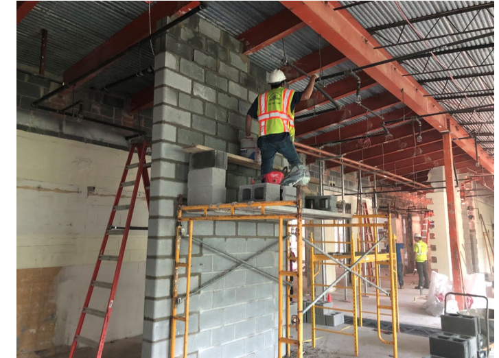
Shoring up building systems in cafeteria area
