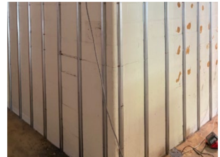
Framing preparation to install drywall over CMU
