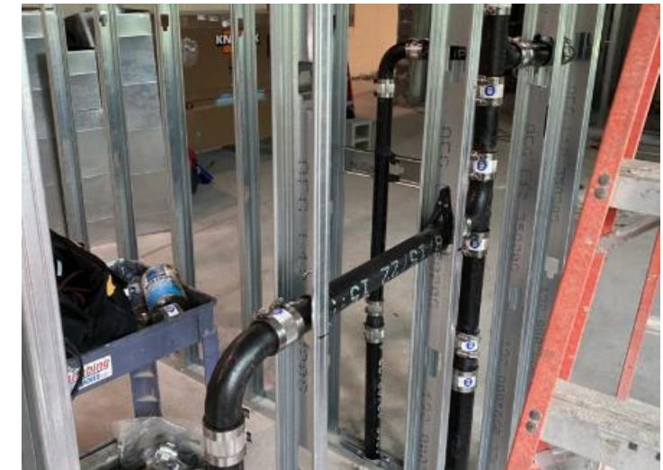
Framing and Plumbing Rough-In
