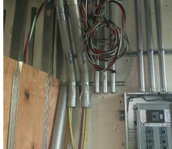
Wire Pull in Kitchen Electronic Closet
