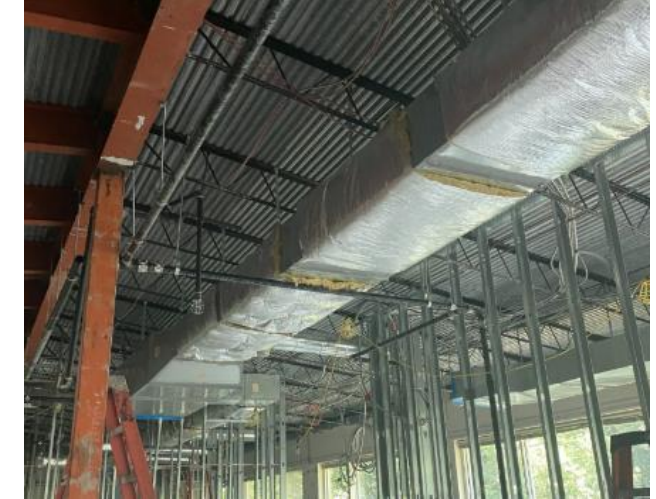
Ductwork installation in kitchen area
